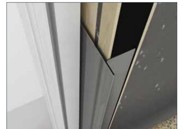
**NOTE!** If using unpainted aluminium in connection with fibre cement products, be aware of surface oxidation.
