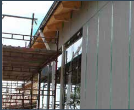
Cembrit Windstopper Extreme has been designed for use as a sheathing board in rainscreen cladding applications
